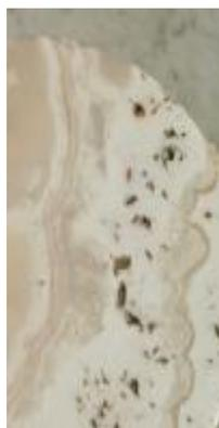
**Figs.144-147** Display the form of small pits - are caused by biogenically induced corrosion processes, particularly in carbonate rocks , it is noticed only on the Egyptian alabaster surfaces of Muhammad Ali Mosque , it is not noticed on the surfaces of chapels at Karnak
