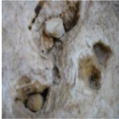
**Figs 67-68** display the third type of vugs and open spaces is large 30-80 cm. long into which protrude almost spherical surface of the travertine of chapels at Karnak of Wadi El-Assiuty
