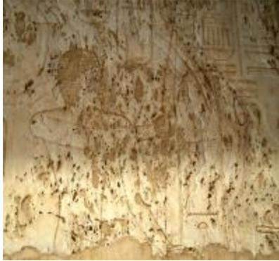
**Figs 65-66** display the first type of vugs and open spaces is a minute cavities of distribution throughout the surfaces of the travertine of chapels at Karnak of Wadi El-Assiuty, and they were stained with red iron-oxide
