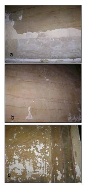
Fig. 3 shows the deterioration phenomena of the imitated marble, (a) shows the missing parts, (b) the arrow points to the crack and (c) shows the exfoliation of the veined layers
