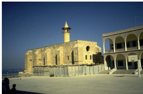
FIG.19 The restored exterior.
