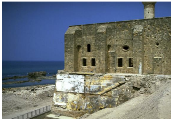
FIG.14 Restoring the hillside on which the building stands
