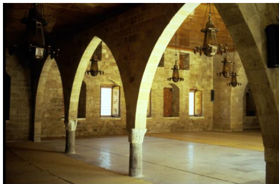
FIG.18 The restored interior .
